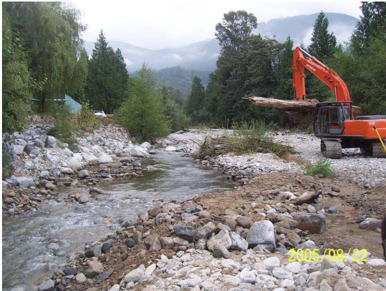
Photograph 9. Upstream of the Anderson property, channel diversions successfully isolated the work area.
