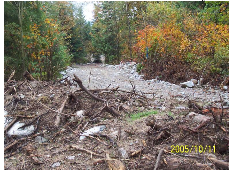
Photograph 15. A berm was constructed to separate Pattison Creek from the right bank haul road on Reach 6. The road was roughened up an alder seed mix applied.
