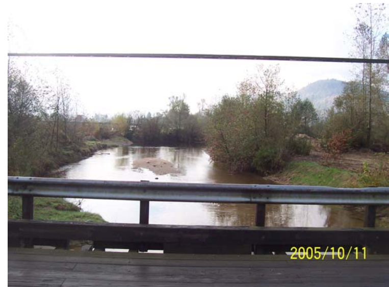
Photograph 16. View downstream of Dale Road bridge. An elevated mid channel bar is forming.
