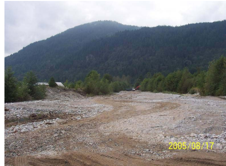
Photograph 7. Looking downstream at the Anderson site after all flow has been diverted to the left bank. The braided channels are dry.
