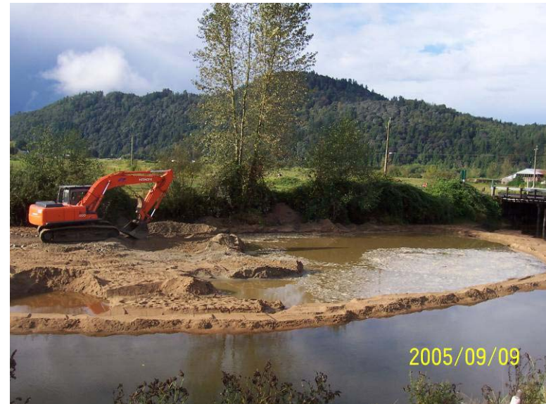
Photograph 4. Excavating the sandbar along the right bank in isolation of flow.
