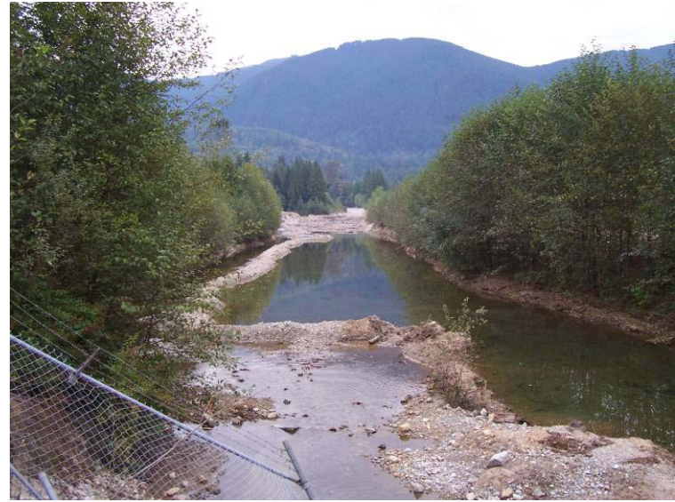
Photograph 19. Looking upstream from Farms Road bridge after excavation was complete. September 14, 2005
