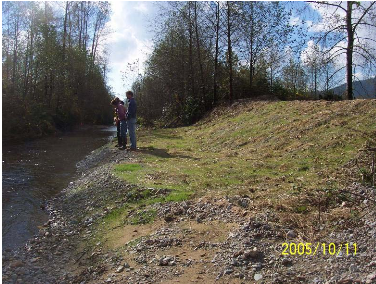
Photograph 21. Looking downstream at the diversion area after the berm and culvert have been removed. Grass seed has taken and the banks are stable.
