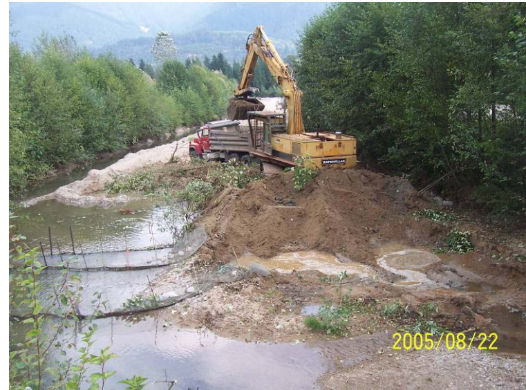
Photograph 11. Removal of the vegetated bar in isolation of flow.
