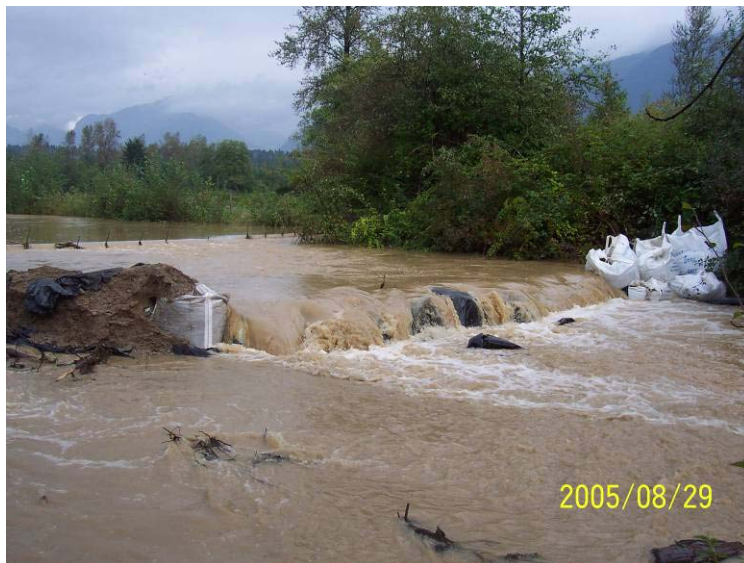
Photograph 10. On August 29, a summer rain event overtopped the berm (as was planned to prevent flooding in the diversion channel) and blew out fish fences.
