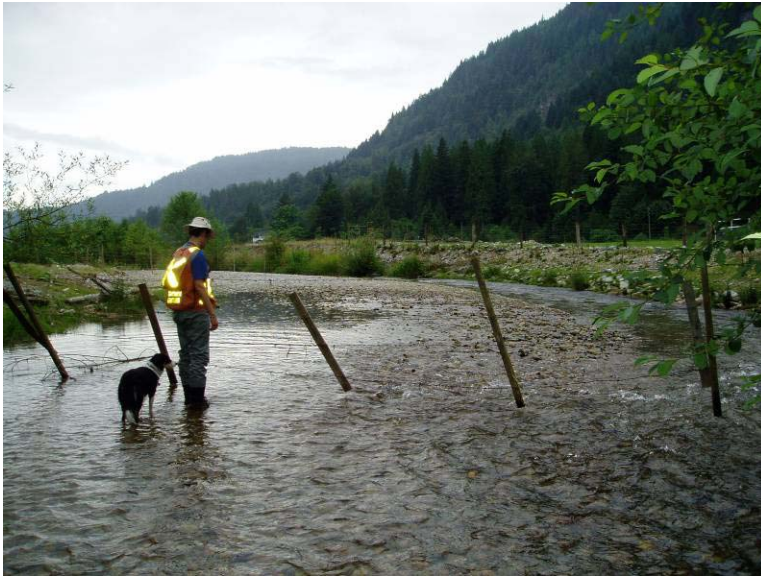
Photograph 1. Looking downstream at the elevated left bank sandbar at Schroots corner prior to excavation. July, 2005.
