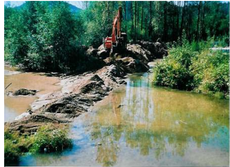
Photograph 3. Sandbags wrapped in a poly liner as well as substrate were used to divert water to the excavated right bank diversion channel. September 6, 2005.
