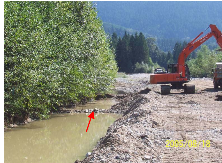
Photograph 8. Once water had been diverted to the left bank a deep channel was excavated along the right bank. Rock weirs were placed to settle out sediment laden water.
