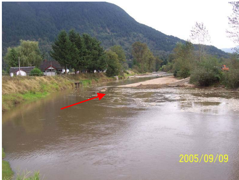
Photograph 5. Water level when the diversion berm in Reach 1 at Dale Road was pulled. Raised water inundated the isolation berms (red arrow). Excavators halted work until levels dropped.
