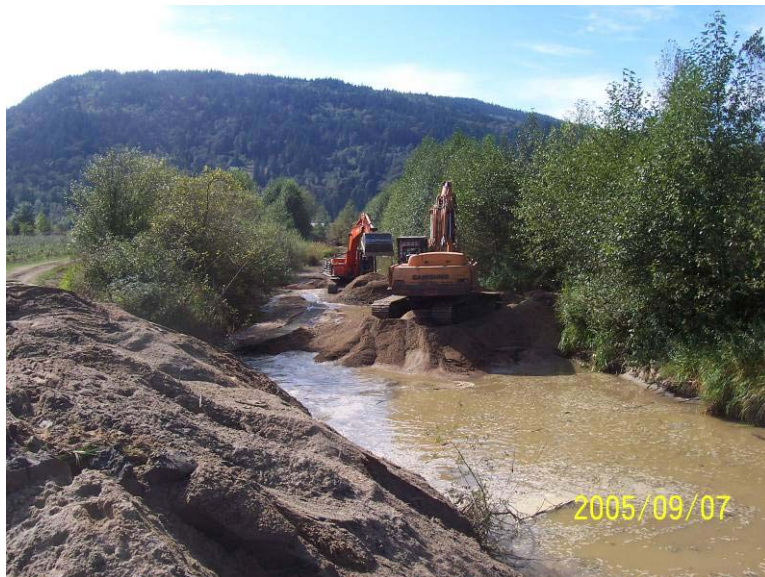
Photograph 5. Excavators worked in tandem in isolation of flow to hoe chuck material to openings in the riparian zone (material placed in the foreground is located at the opening in Photograph 2).
