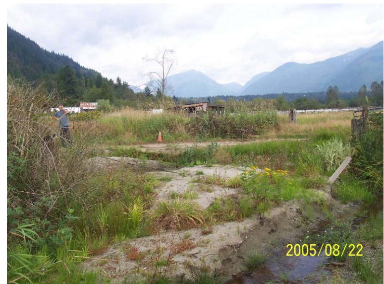
Photograph 4. The Bouchier Creek channel required excavating prior to flow diversion from Lagace Creek. The channel had filled in and blocked a culvert due to a debris torrent.
