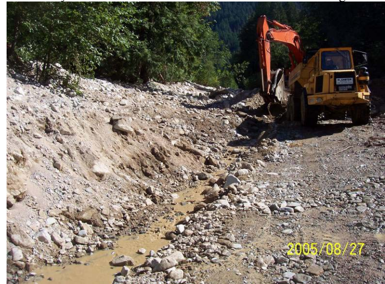
Photograph 11. During gravel excavation and recontouring, water seeped into the isolation site. Water was directed into a shallow swale.
