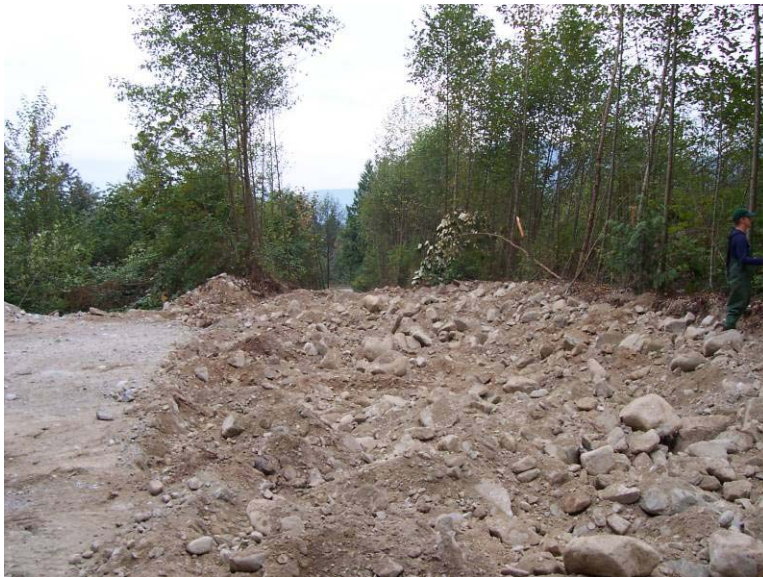
Photograph 14. The haul road along the left bank was decompacted and an alder seed mix applied. Compacted gravel to the left of the photograph will be removed by the landowner. September 14, 2005.
