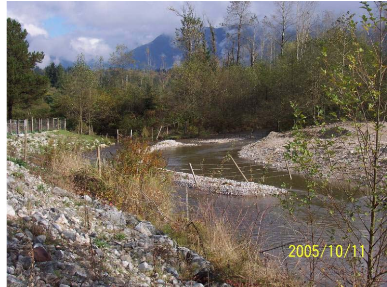
Photograph 19. The left bank sandbar at Schroots corner with berms breached at completion of works. Temporary spoil piles have been removed.
