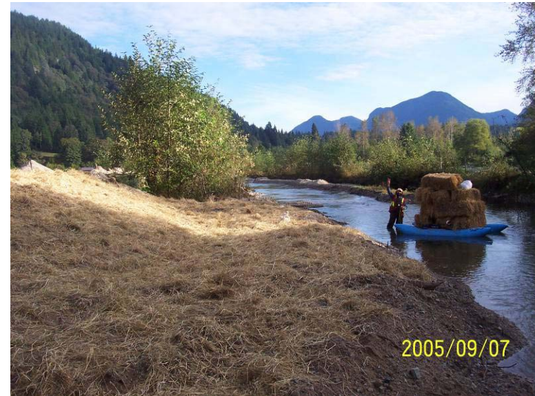
Photograph 11. Looking upstream at the diversion area after the berm and culvert have been removed. The site is stable, seeded and covered with straw.
