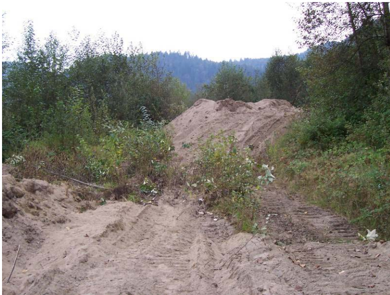
Photograph 10. View of temporary spoil pile placed on the access road on the west side of Lagace Creek.
