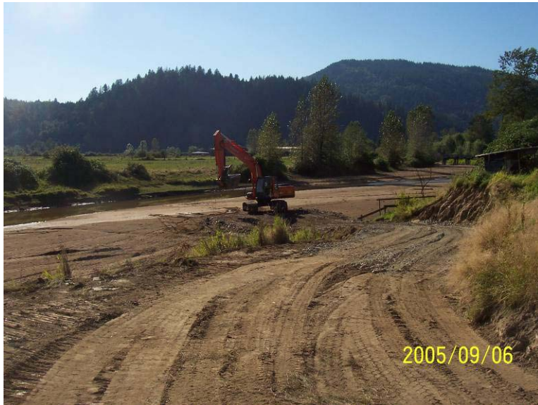
Photograph 1. Looking at the upstream sandbar and access along the left bank at commencement of work. In the background, the right bank sand bar can also be seen.
