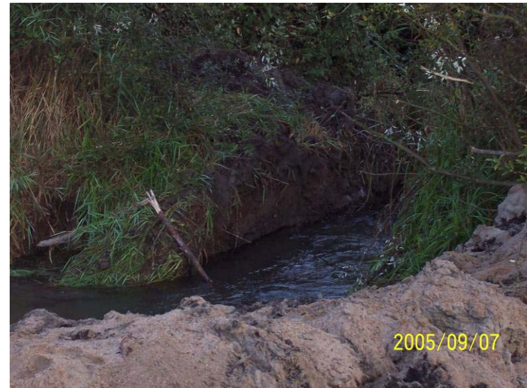
Photograph 4. A substrate berm was placed directly upstream of the diversion outlet effectively isolating the 300m excavation area. Pumps were not needed in the isolated excavation area.
