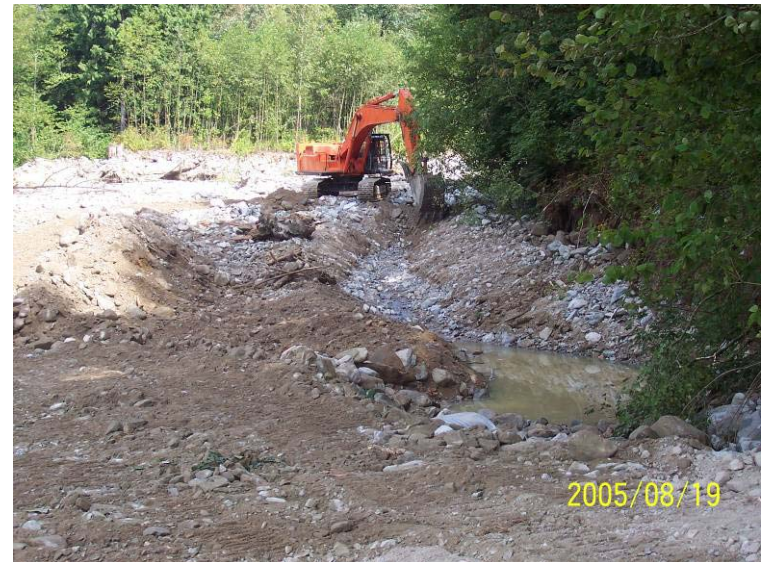
Photograph 8. In order to work in the dry, all flow in Reach 6 was diverted to an excavated channel along the left bank.
