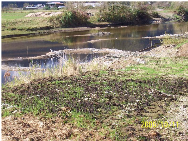
Photograph 6. Looking upstream at the excavated sandbar and access along the left bank (see Photograph 1). Grass is growing, berms are breached and the site is stable.
