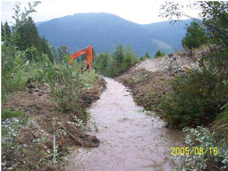
Photograph 6. The left bank channel was deepened in spots to direct water away from the right bank. This caused sediment plumes for up to 45 minutes in duration.
