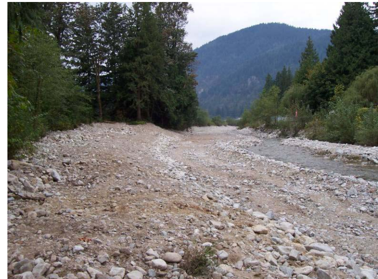
Photograph 16. Looking downstream from Seux Road Bridge at completion of the work. September 14, 2005
