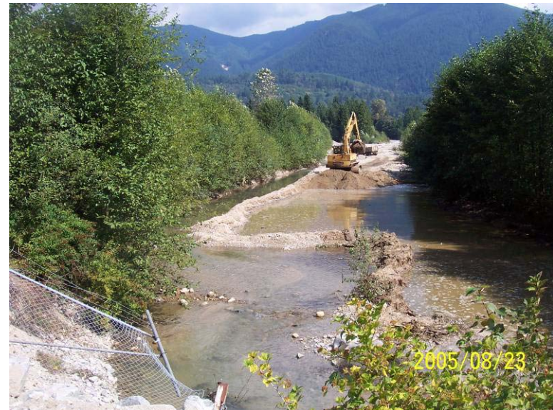
Photograph 12. Excavation in isolation of flow.
