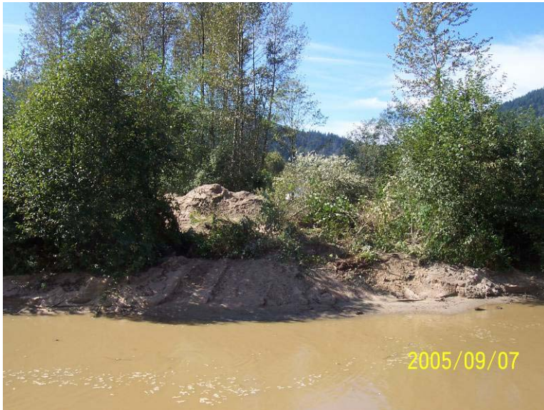
Photograph 13. Looking at the right bank at an opening used to spoil material onto the eastern access road. Riparian vegetation was salvaged and replaced.
