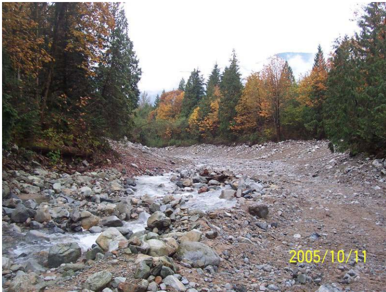
Photograph 18. View of Reach 6 in October from the upstream end of the flood protection works.
