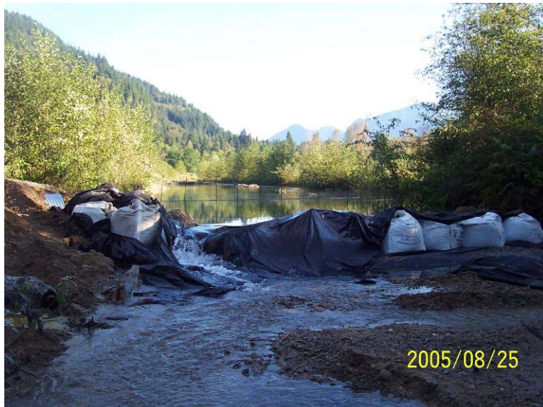
Photograph 6. Reduced flow was maintained throughout the excavation, as salvage operations were occurring concurrently directly upstream of the excavation operations.
