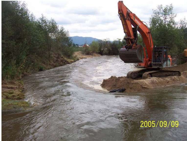
Photograph 9. Once excavation works were completed, the dam was breached and the diversion channel filled in. The dam breach caused isolation areas in Reach 1 at Farms Road to fail.
