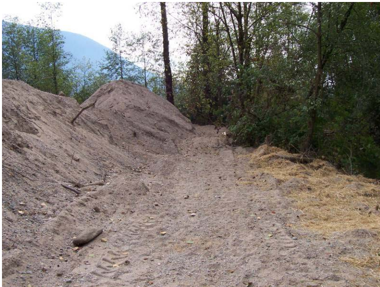
Photograph 14. View of temporary spoil piles along the left bank. A bench was created to separate the spoil from the sloped river bank (straw covered area).
