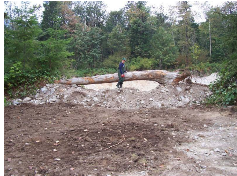
Photograph 16. View of Reach 5 access at completion of work. The access has been seeded.
