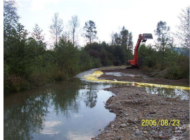
Photograph 3. Excavating a right bank sandbar between Schroots corner and the diversion using the Megasecure and berms to divert flow.
