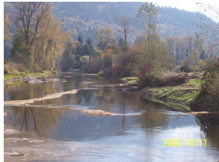
Photograph 8. Looking downstream from Farms Road Bridge. At the right bank excavation (Photographs 3 and 4). Berms are breached and grass is growing on the banks.
