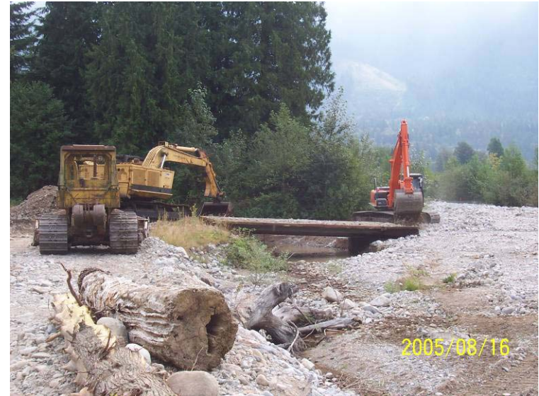
Photograph 3. Placement of the bridge at Andersons site to access the bar.
