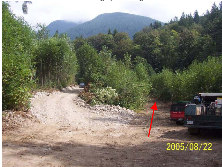
Photograph 9. View of the completed haul road. Cleared vegetation to the west (red arrow) was outside the 30m setback and was used to store gravel
