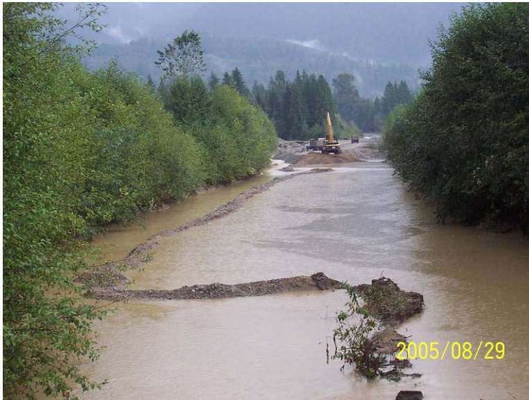
Photograph 13. Rain event on August 29.
