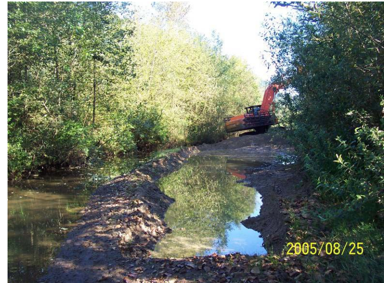
Photograph 7. Once isolated, excavation between 302 and 460m from Schroots Corner took place by scalping isolated bars. Bars were only scalped to approximately 0.45m to encourage fall spawning.
