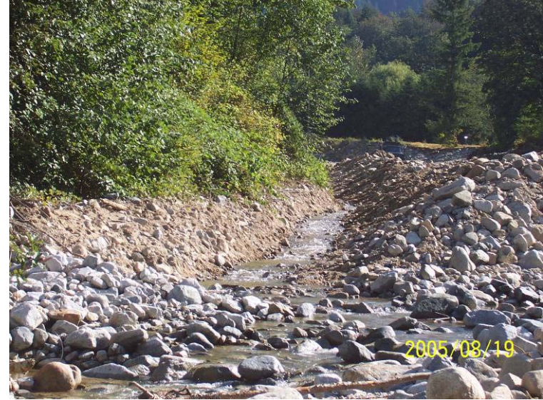
Photograph 7. In order to work in the dry, all flow in Reach 5 was diverted to an excavated channel along the right bank. Flow was diverted away from the right bank near the bridge to conduct right bank stabilization work.
