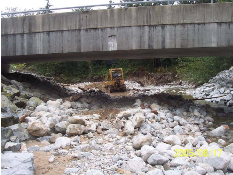
Photograph 5. A small bulldozer was used to grade the gravel bar to allow access for a D8. The D8 forded the channel several times to access and prep the upper portion of Reach 6.
