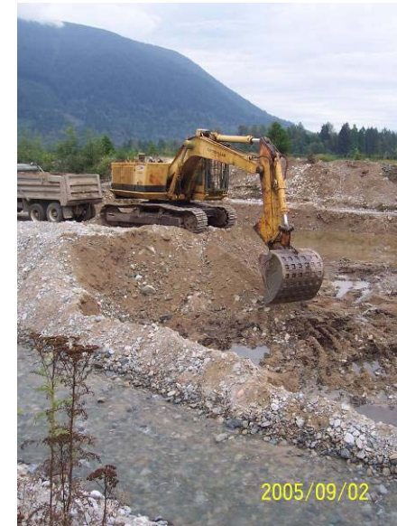
Photograph 15. At approximately 2/3 of the way upstream to the temporary bridge crossing, excavation was almost in the “dry” (little flow seeping into the excavation site).
