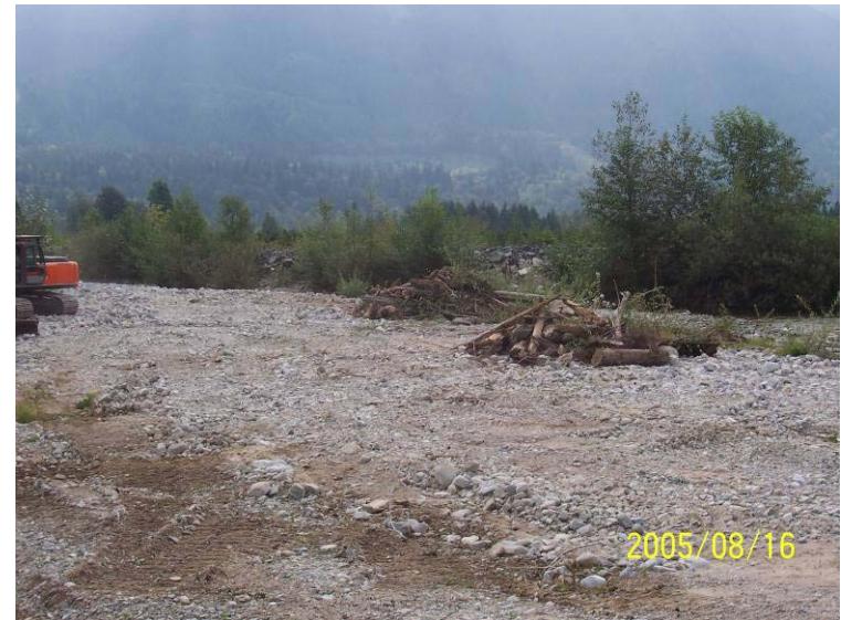
Photograph 4. Woody debris was removed from the bar prior to excavation. Unbeknownst to the on site monitors, anchored in large woody debris was also removed.
