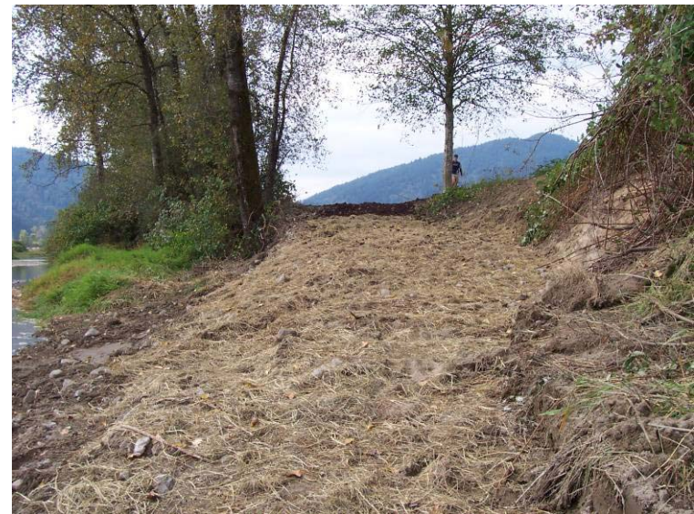
Photograph 7. Looking up at the second access road along the left bank of Lower Reach 1 upon completion of work. The access has been seeded and both straw and silage applied. September 13, 2005.
