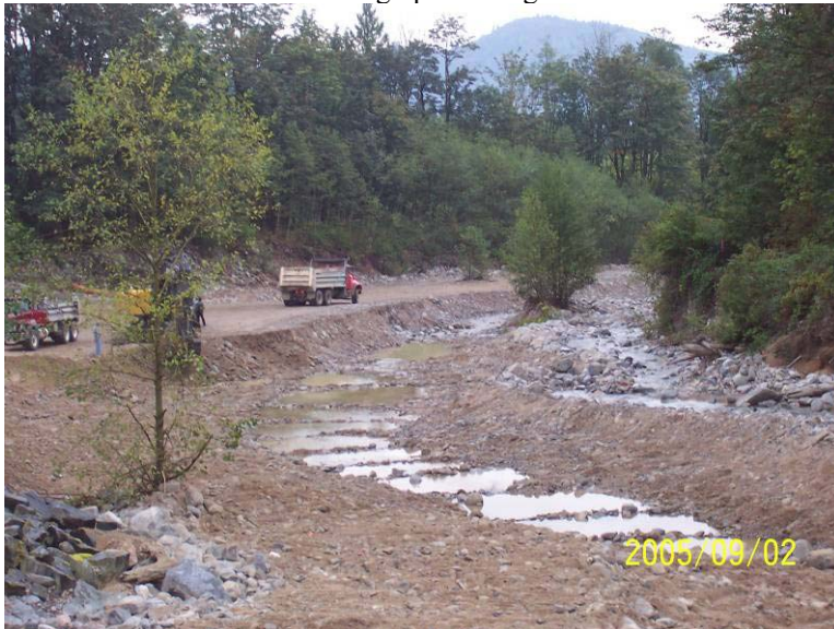
Photograph 13. A series of sediment traps were excavated to settle out seepage water in the excavation site within Reach 5.
