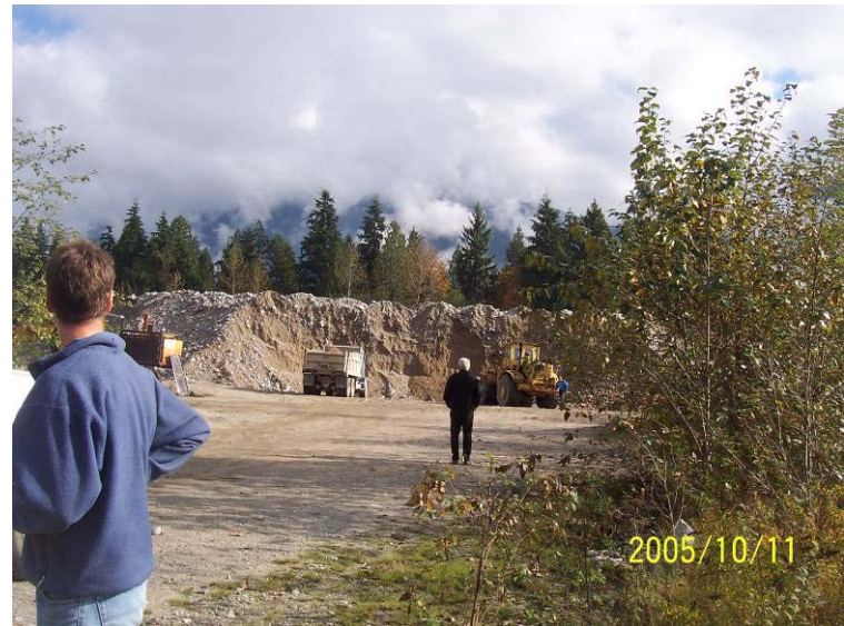
Photograph 20. View of excavation spoil pile on Anderson's property.
