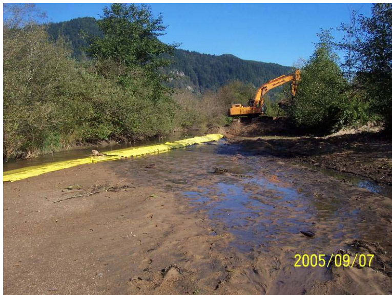
Photograph 6. Megasecure was used in two locations in Reach 1 to enable extraction of sandbars on the left bank in isolation of flow.
