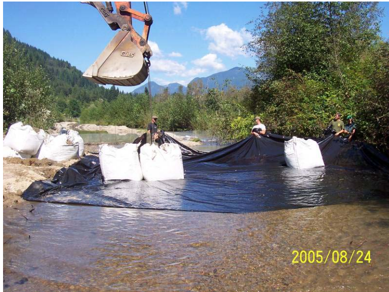
Photograph 5. Sandbags wrapped in a poly liner were used to divert water to the excavated right bank diversion channel. Some substrate was also used on the upstream side to ensure a proper seal.
