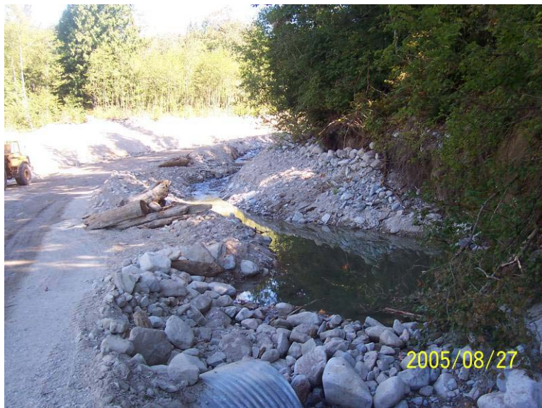
Photograph 10. View of completed diversion channel along the left bank of Reach 6.
