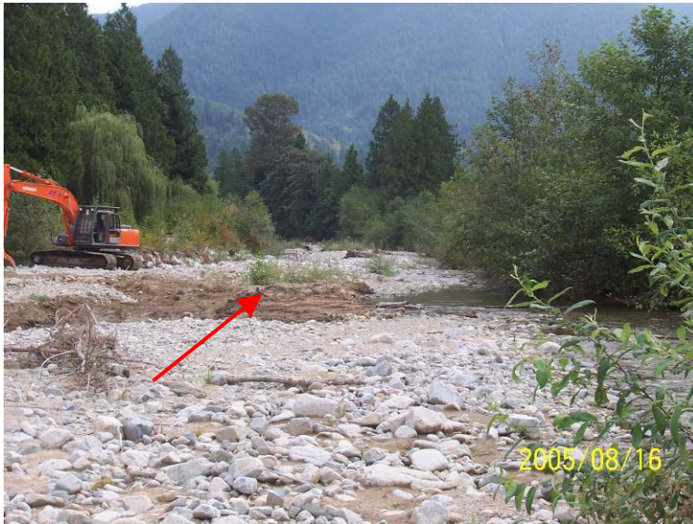
Photograph 5. All flow was directed at to the left bank by berming the intake of small seepage channels to the right bank
