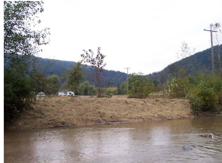
Photograph 11. Looking west at the diversion dam location after the site has been seeded, covered with straw and vegetation replaced at the top of the bank.
