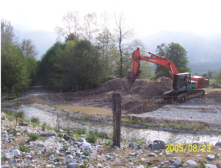
Photograph 2. The left bank sandbar at Schroots corner being excavated in isolation of flow.
