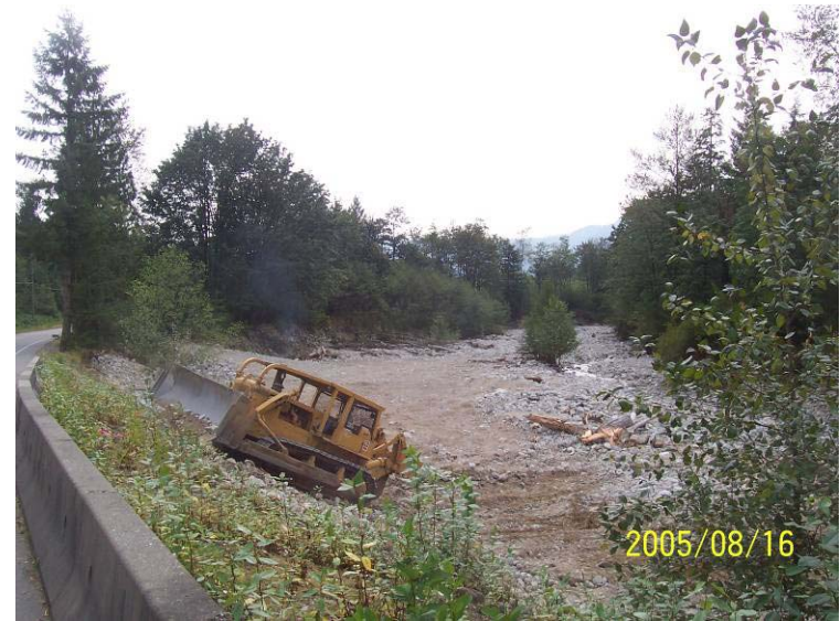
Photograph 4. Looking downstream at Reach 5 from Sylvester Road bridge at the inception of recontouring and bank stabilization in isolation of flow.
