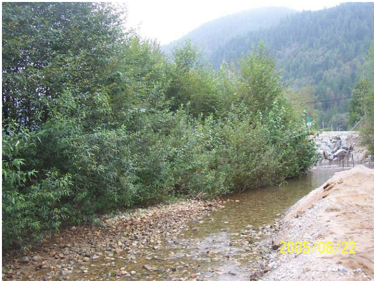
Photograph 10. View of 38 by 5m vegetated bar that was removed in order to direct flows away from the eroding right bank near Farms Road bridge
