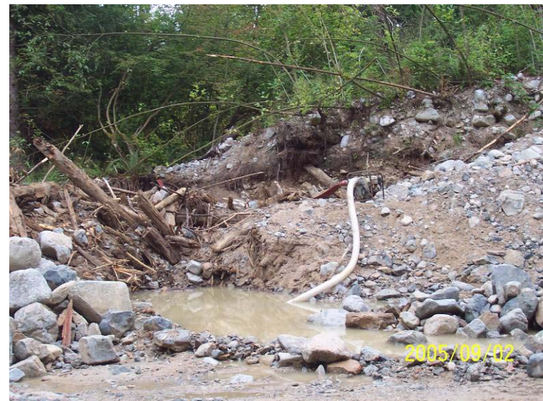
Photograph 12. Water from the shallow swale entered a sediment trap and was pumped out using a 3" pump.
